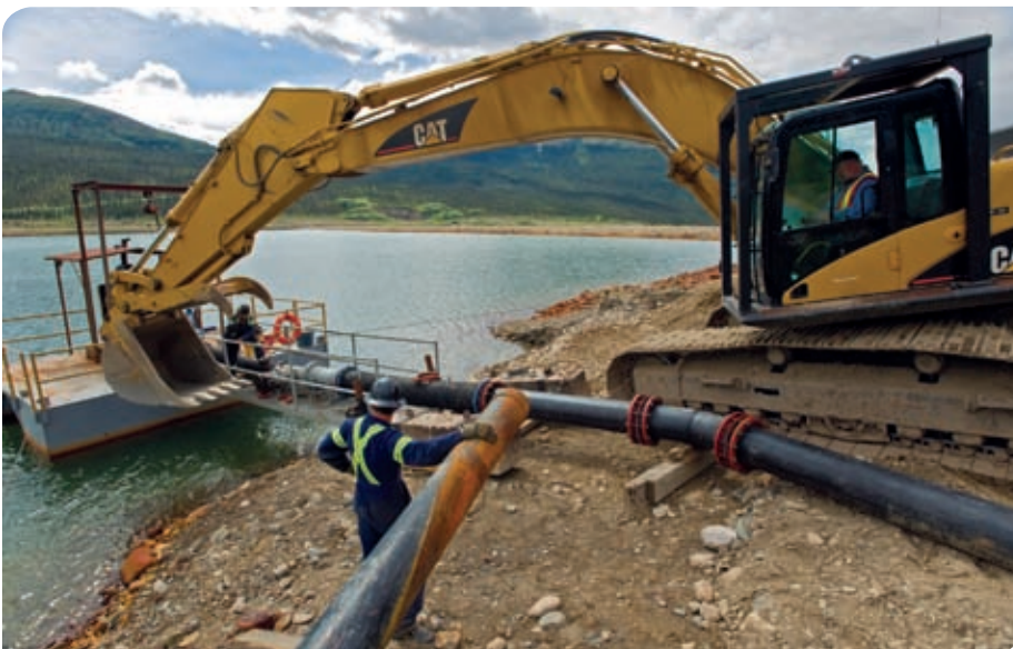
Pipe installation at the Intermediate Pond Barge
