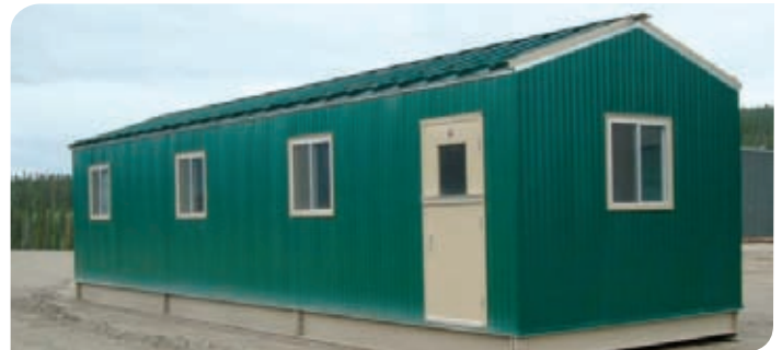
The new analytical lab on site at the Faro Mine Complex.
