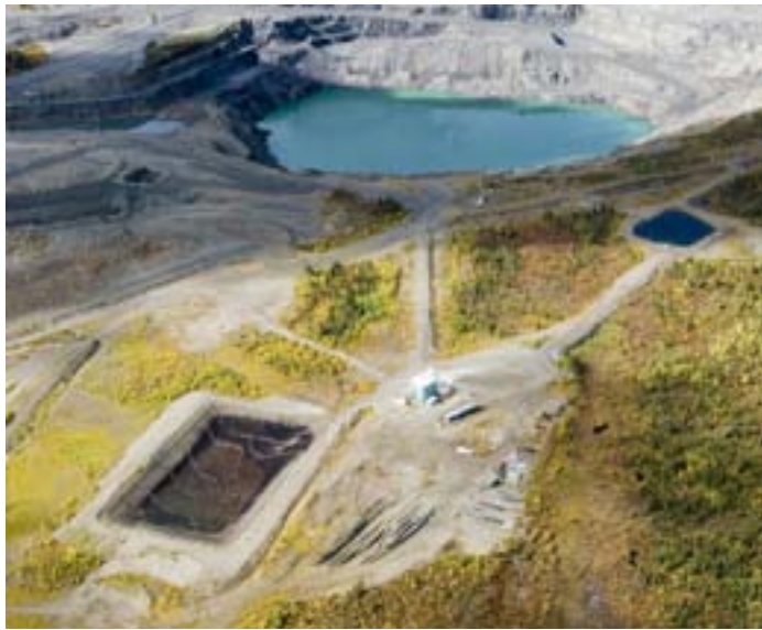
Grum pit and water treatment plant.
