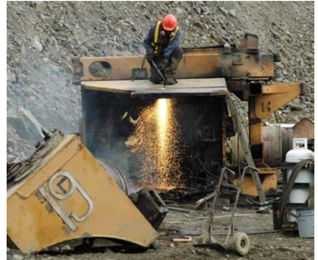
Abandoned machinery is cut down to scrap metal for removal from the Faro Mine complex as part of site remediation.
